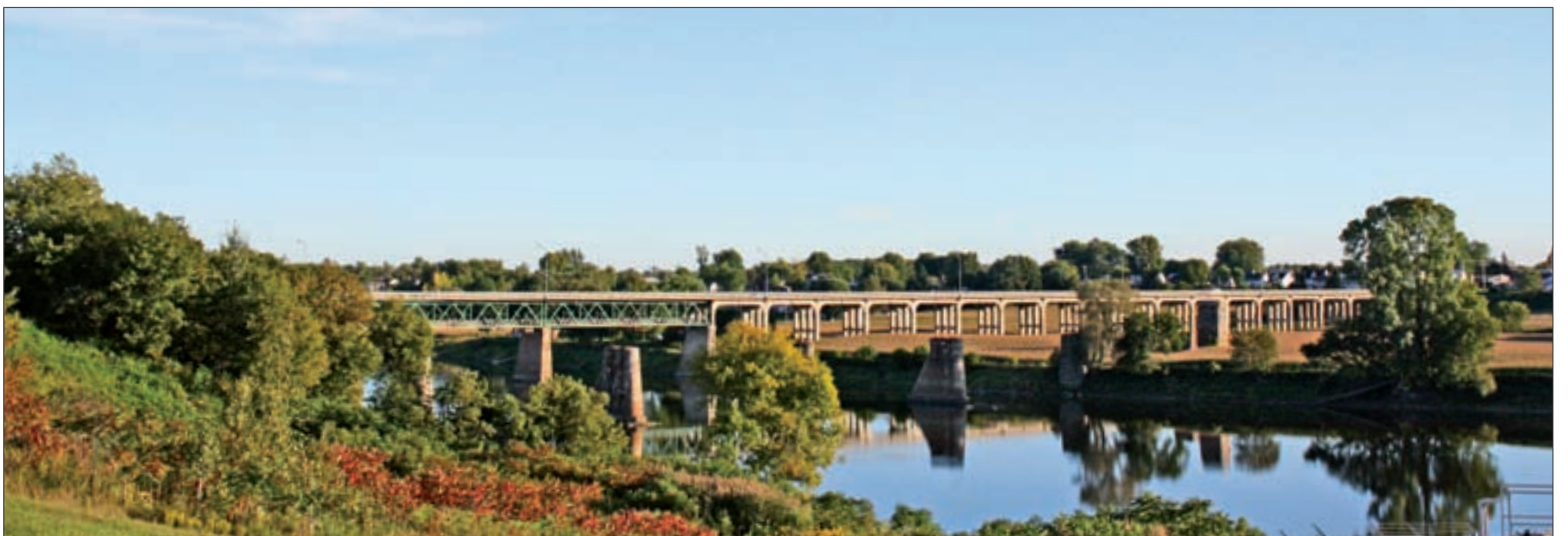
David-Laperrière bridge, viewed from the Community Centre M8WIGAMIKW.
